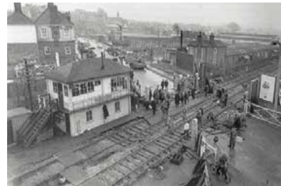
A view of the signal box in 1968
