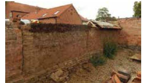
Section of wall during repairs (image courtesy of Nottinghamshire County Council)
