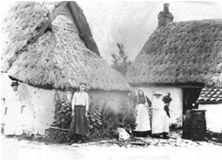
Mud cottages of Little Lunnon (image courtesy of Nottinghamshire County Council)
