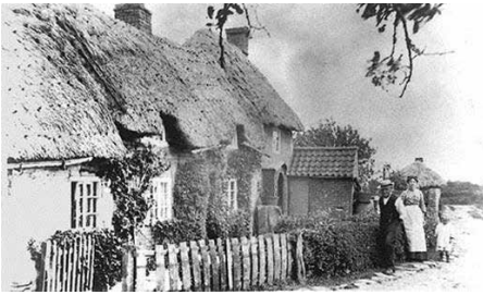
Mud cottages of Little Lunnon (image courtesy of Nottinghamshire County Council)
