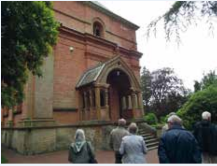
The tour moves on to the entrance to the pumping station
