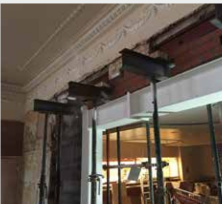
New steelwork and original Victorian detailing
