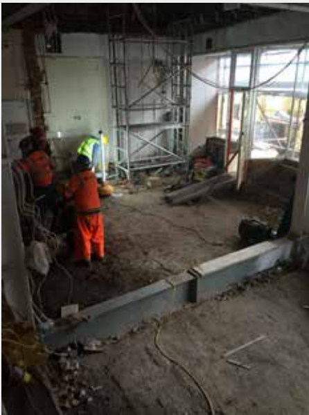
The installation of the new steel beams and columns
