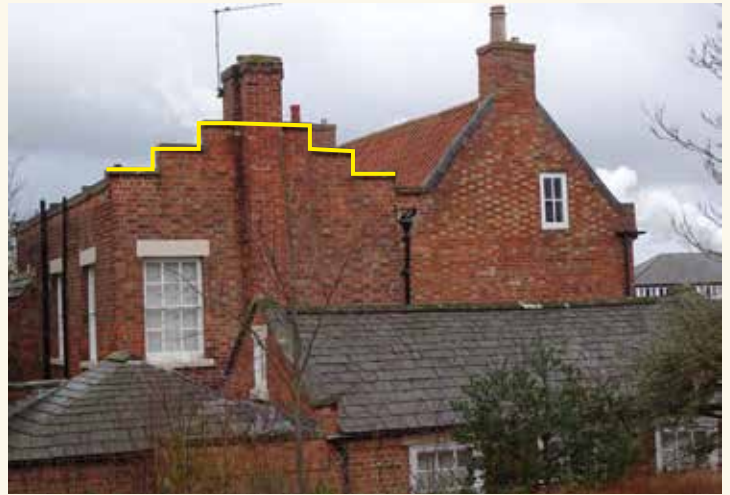
Crowstep Gable at the former Toll House, Beastmarket Hill
