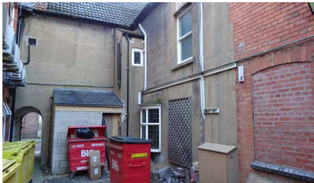
Rear of the property during refurbishment
