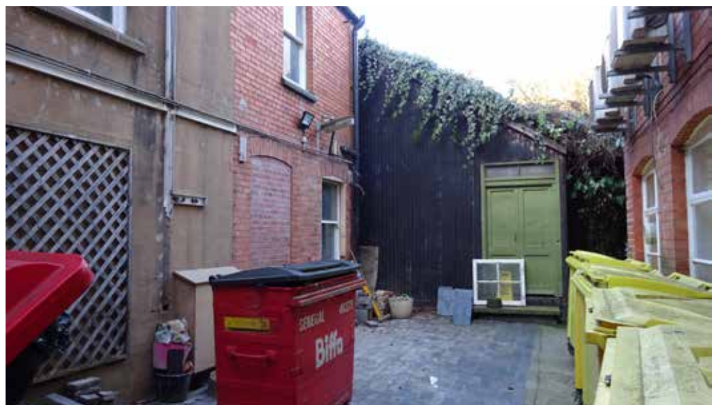
Rear courtyard and post-war warehouse, the dentist surgery is to the right
