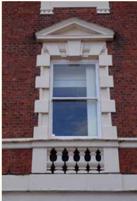
Gibbs Surround to first floor window of the Clinton Arms
