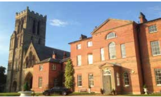
The Priory and Georgian mansion today
