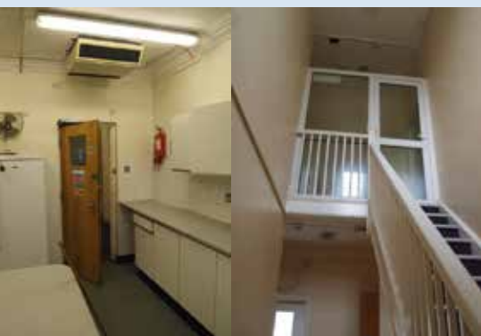
Previous internal modifications and alterations
